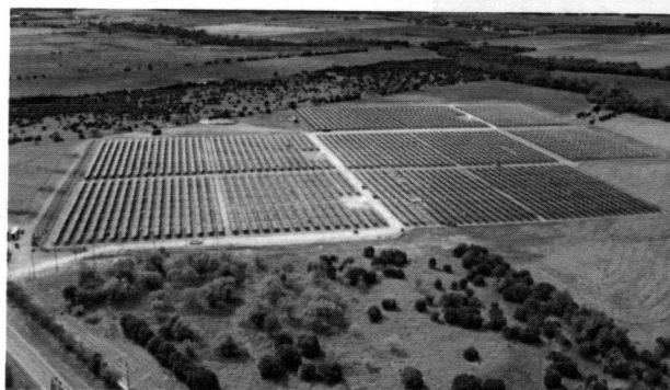
▲ Walnut Springs, Walnut Springs, Texas, 7 MW
